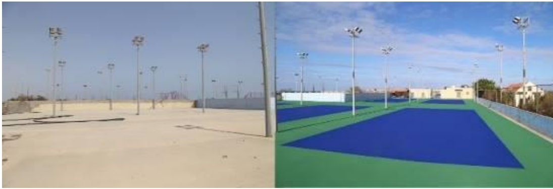
The tennis court before and after the rehabilitation in Sabratha. ©UNDP Libya
